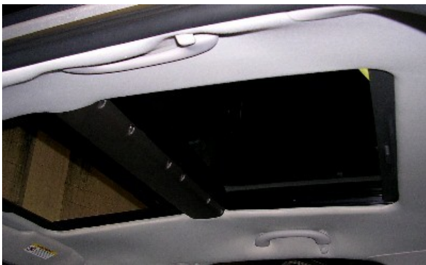
Handles and visors keep the headliner taut. Note the interior cross piece in the sunroof that hides the motor and wiring. It's the same color as the sun shades which can be closed even when the glass panel is open, blocking any wind and buffeting. The shade is mesh so some light always comes through the sunroof even when the shades are closed.
