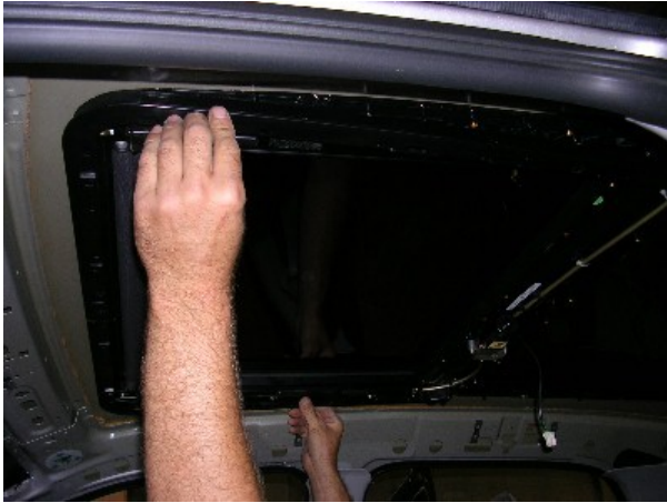
Tracy screws in the interior framework which pulls the exterior frame closer to the CV's roof, squeezing out the silicone.
